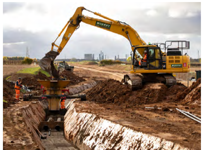
Backfilling a trench with cable ducts laid (Sofia Offshore Wind Farm)
